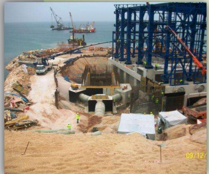
RETURN LINE (ENTRANCE OF JET CHAMBER)
