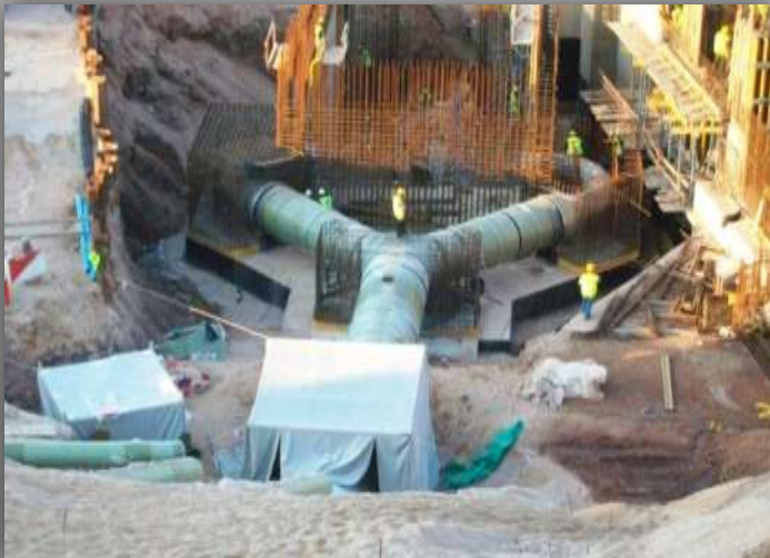
RETURN LINE (ENTRANCE OF JET CHAMBER)
